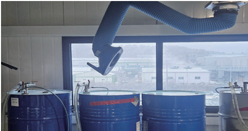
Installation of an arm hood in the measuring room
