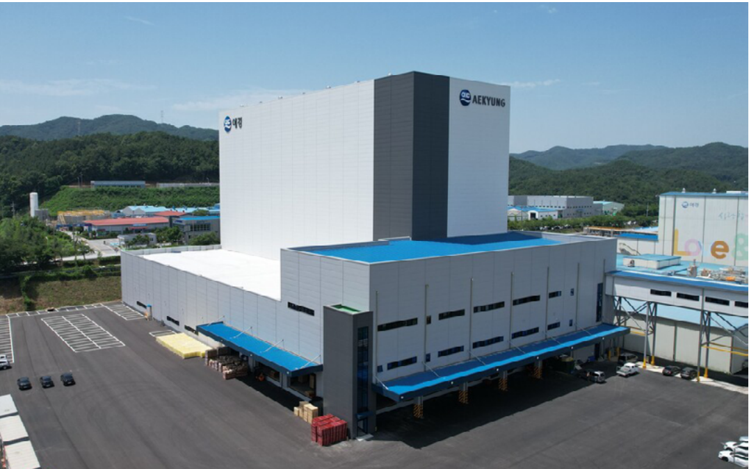
2023 - Aekyung Industrial Central Distribution Center (AK CDC)
