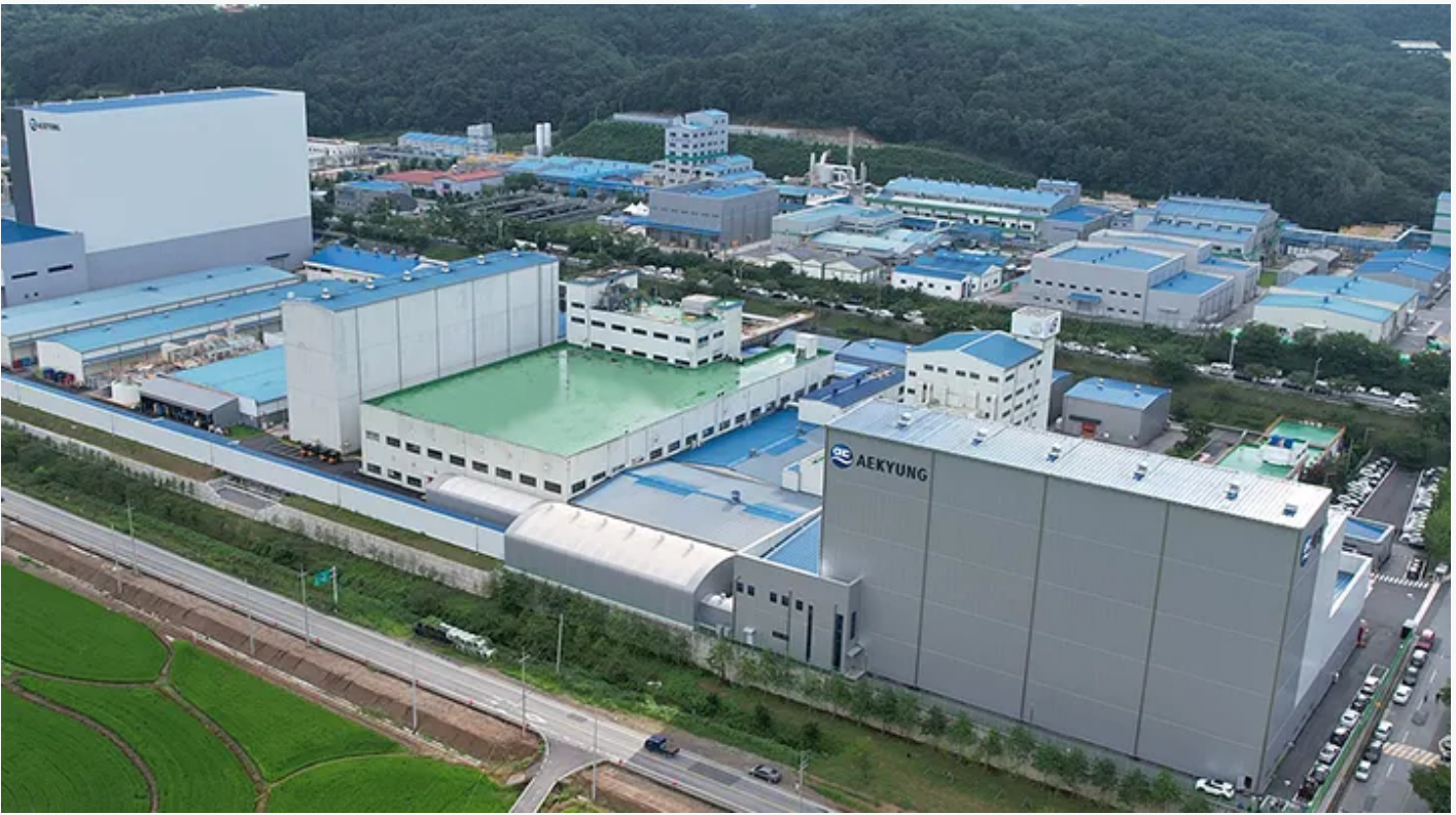
Aekyung Industrial Cheongyang Plant
